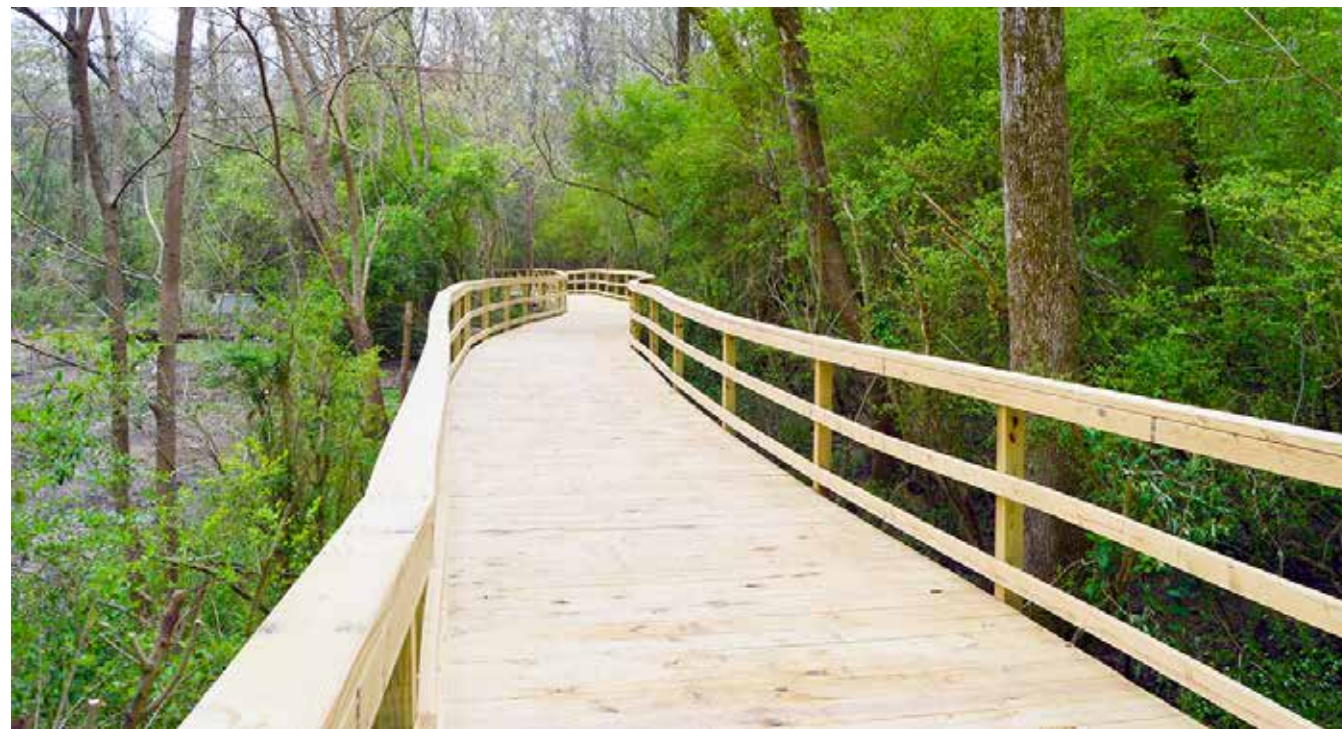
ABOVE A new boardwalk installed as part of the trail network around Rosel Fann Recreation Center in 2016.
